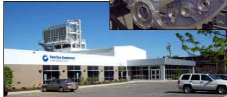
11 th Street Facility - Engine Systems
